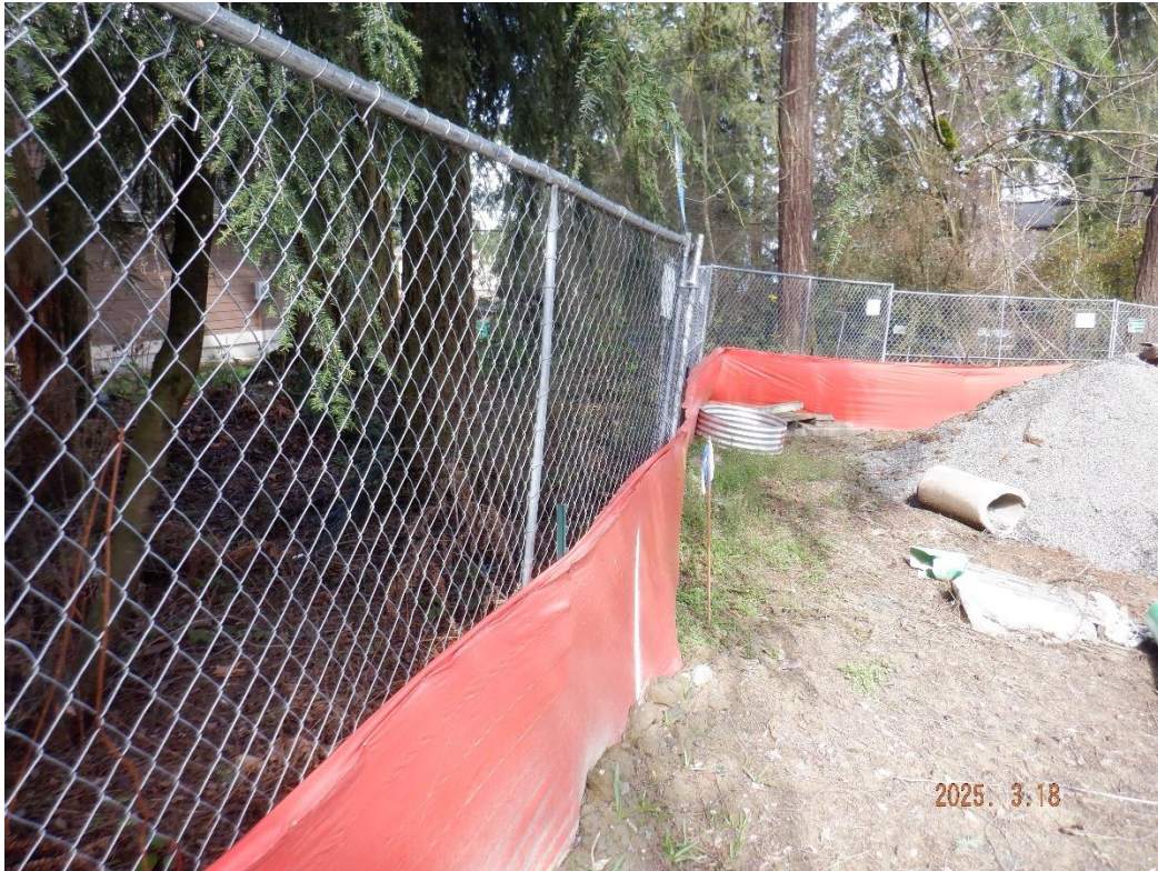
Tree Protection Fence adjacent to Tree #4
