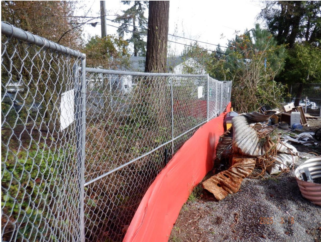
Tree Protection fence positioned roughly 5-feet from trunk face of #1
